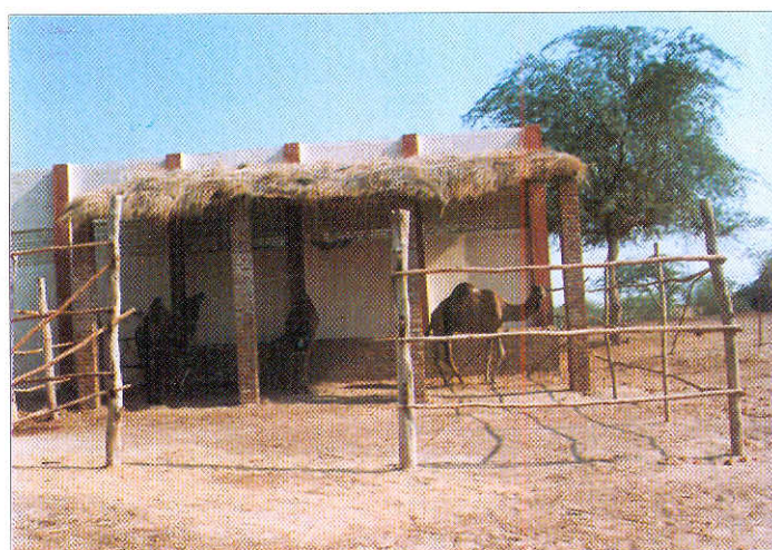
Fig. 4.6.4.1 Thatched roofed open type kachcha shelter
