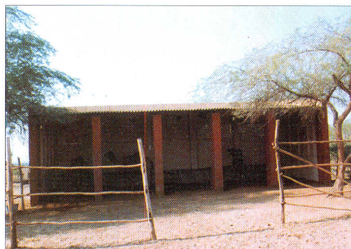
Fig. 4.6.4.2 Asbestos roofed close type concrete shelter
